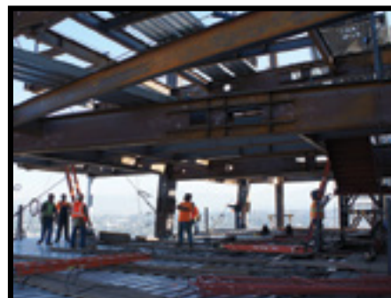
Structural Steel Erection
